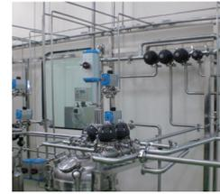
Distribution loop pipings manufactured by us which are used to connect the main water equipment, tanks, skid, pumps, heat exchangers and point of usage (POU) in one closed circuit system with piping and valves
