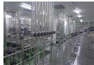
Distribution loop pipings manufactured by us which are used to connect the mixing vessels, storage tanks, filters, CIP/SIP and pumps into one closed circuit system with piping and valves.
